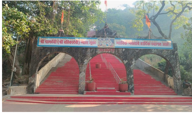
The front stairway to the temple
