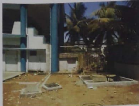
RING WELL WITH FLUSH VALVE CHAMBER
