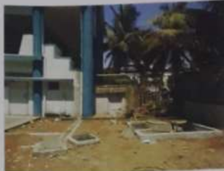
RING WELL WITH FLUSH VALVE CHAMBER
